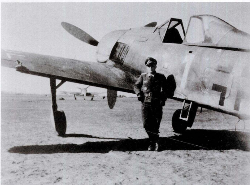
LEFT: Hptm. Helmut Wettstein, Staffelkapitän of 6./JG 54, with his Fw 190 'White 1' in the Courland pocket. Note the black outline style Balkenkreuz on the fuselage and blown canopy which made it possible to install the type of head armour shown.
