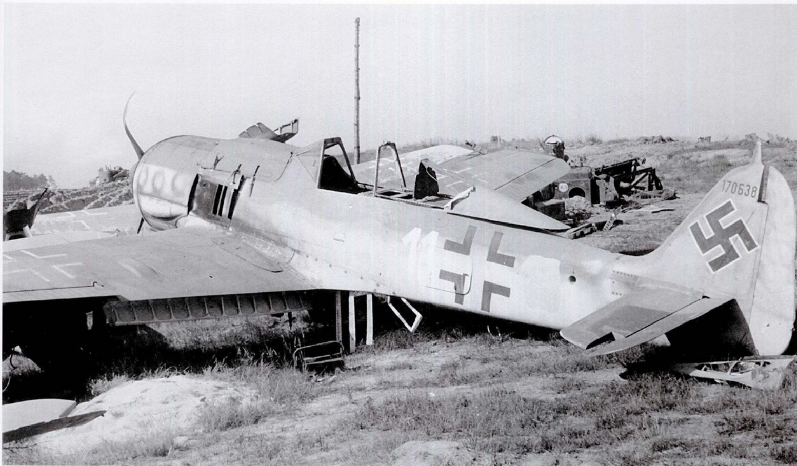
ABOVE: 'White 11' was found abandoned at Berlin-Gatow at the end of the war but was photographed in early 1946. The Werknummer 170638 confirms that this is an Fw 190 A-8 manufactured in October or November 1944 and was probably finished in 81 and 82 on the uppersurfaces with 76 on the fuselage sides and undersurfaces. Both uppersurface colours have weathered and faded so that the new 81 or 83 sprayed over the repairs on the horizontal tail unit and the starboard outer wing show as dark patches against the original colours. Note also that where the tactical number has been moved from behind the fuselage Balkenkreuz, the patch of 76 is possibly the grey-green shade.
